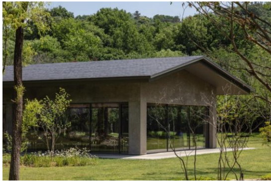
FIG 26 Closer views of the building
