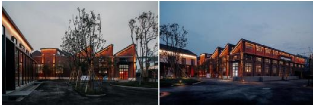
FIG 5 Exterior night view of the building
