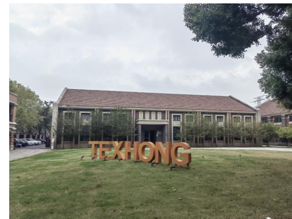
FIG 7 Facade of Building 2 of Daming Yarn Factory in Changzhou
