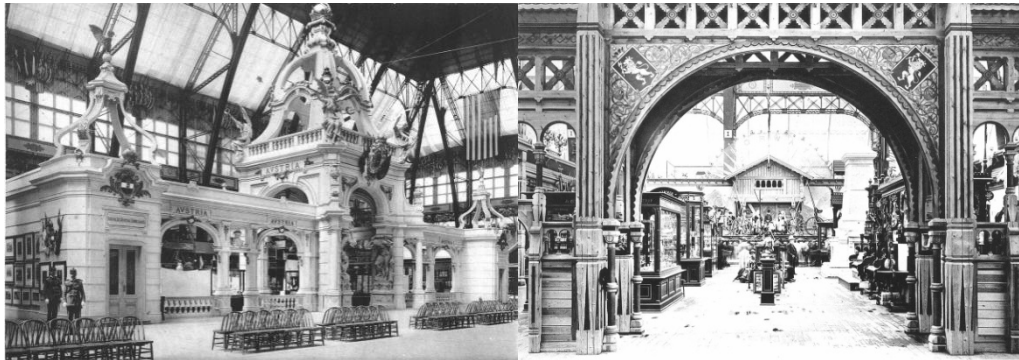
AUSTRIAN EXHIBIT,—MANUFACTURES BUILDING.
