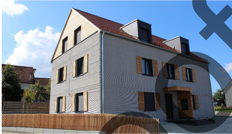
FIGURE 3. House Wallenhausen built using 3D technologies [13].
