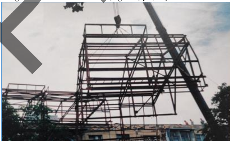
FIGURE 5. Erection of a high-quality bar sections framework over an additional floor. Photo by Tatiana Karzhyneroва
