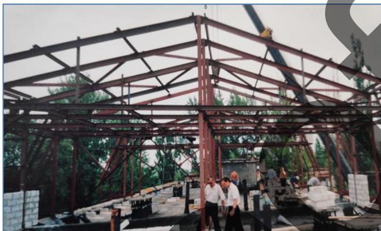
FIGURE 6. Roof trusses and load-bearing structures of building attic erection. Photo by Tatiana Karzhynerova
