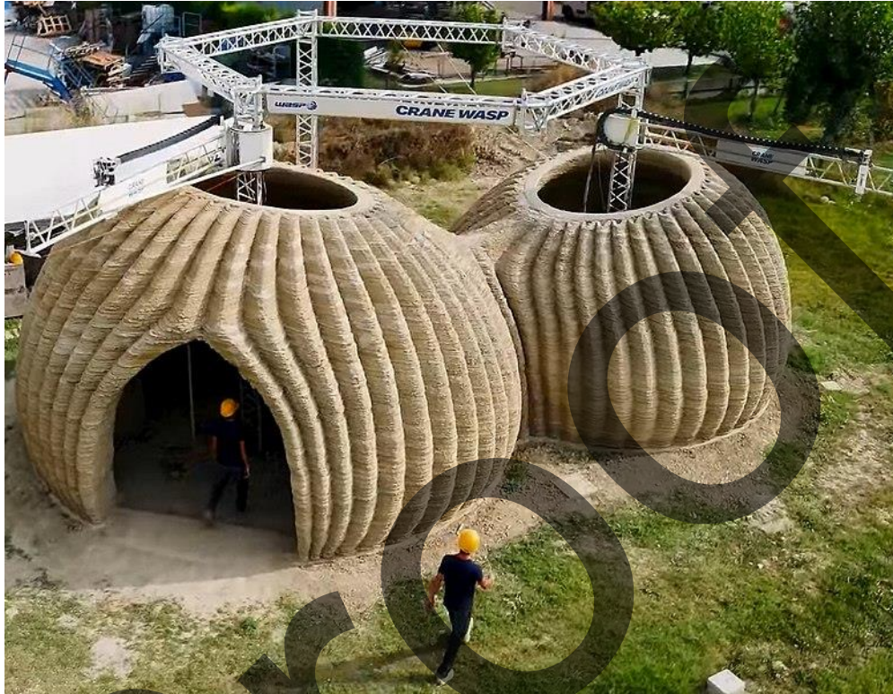
FIGURE 5. Eco-sustainable 3D printed house "Tecla" [18].
