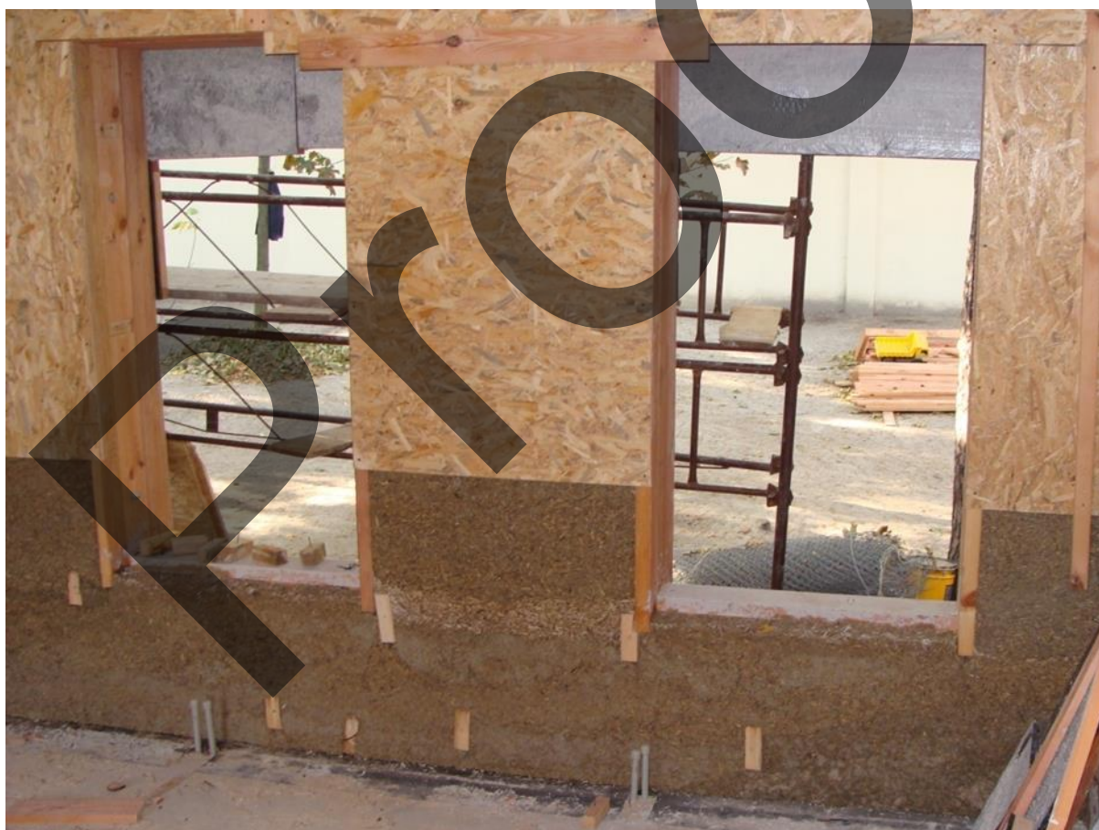
FIGURE 2. Hemp concrete wall, made using monolithic technology
