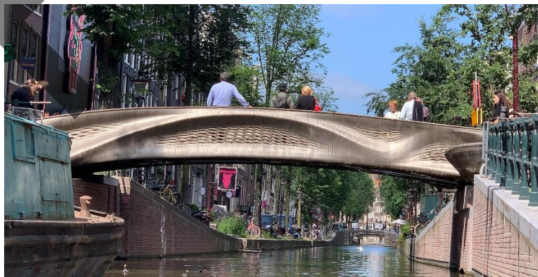
FIGURE 2. Stooftbrug Bridge made on a 3-d printer, Amsterdam [11].
