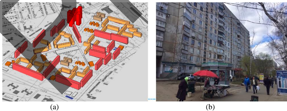
FIGURE 3. Micro-district 605 in Saltivka, Kharkiv, Ukraine, the 1970s: (a) - 3D model; (b) - large-panel 12-storeyed living blocks, typical project II-57 series; source: co-author Oksana Chabanyuk, 2017.
