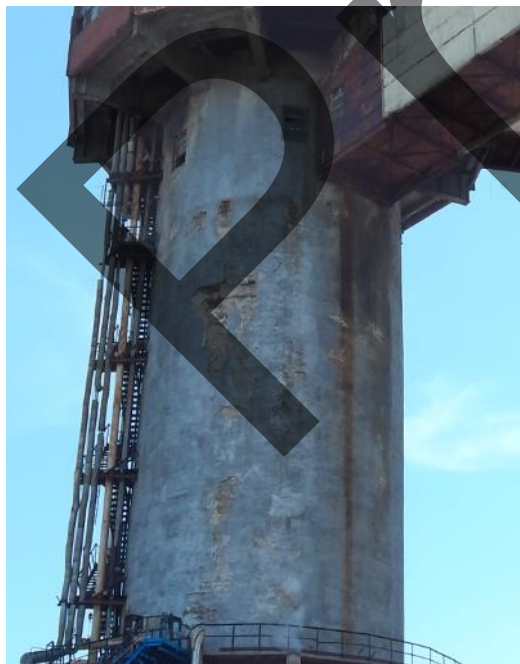
FIGURE 1. The tower trunk with large areas of concrete surface degradation
