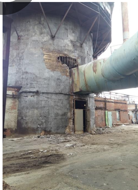
FIGURE 2. Full destruction of trunk, absence of horizontal steel reinforcement
