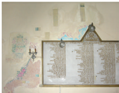
16. Back of Women's Gallery before 2010 restoration work
