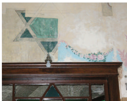
14. Back of Main Sanctuary.
